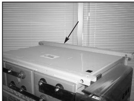
Figure 4: Recommended Frame Ground Location
