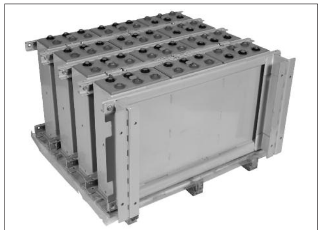
COMPLETED I-BEAM SUPPORT TO MODULE INSTALLATION Figure 10
